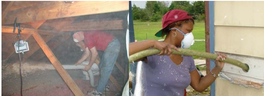
Cellulose insulation is blown into an attic to reduce heat loss
