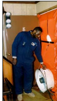
The blower door is used to quantify and locate air leakage
