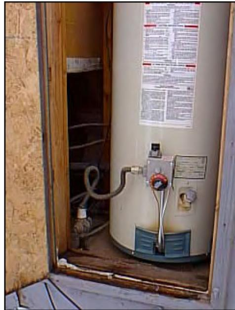
**Mobile home water heater closet with gas-fired water heater**
